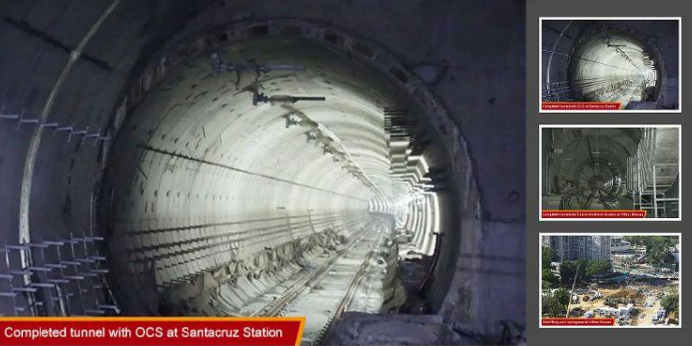
Completed tunnel with OCS at Santacruz Station
